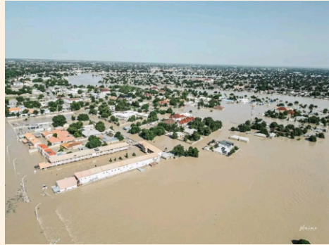
A photo showing houses submerged in the flood waters in Maiduguri.
